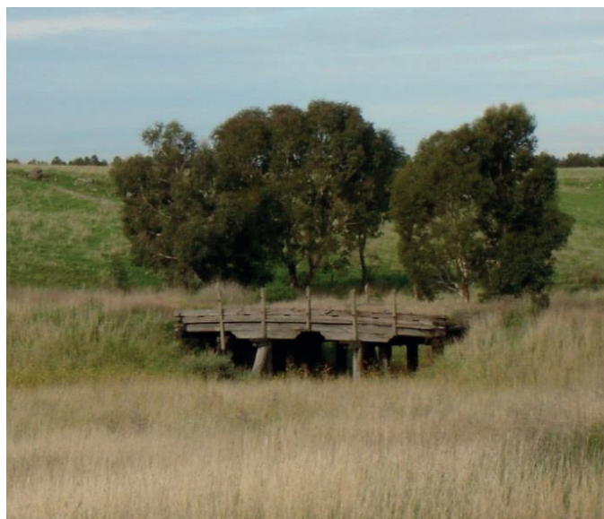
Burchett Creek Bridge (H1856, HO35) on the old Hamilton Highway 2.1 km east of Caramut over the Burchett Creek. Bridge dates to the late 1870s. (Image courtesy of Tardis Archaeology Pty Ltd).
